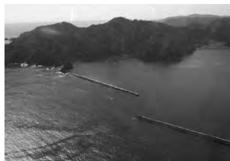
釜石港湾口防波堤
