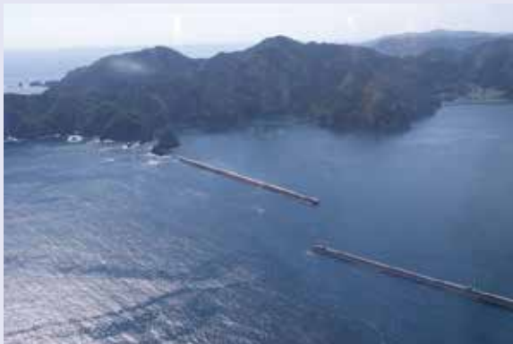
釜石港湾口防波堤
