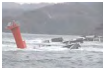
釜石港湾口防波堤
