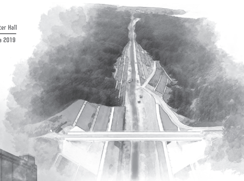
Improvement of National Route 45 at Sakanoshita Iwate, Japan 2020
