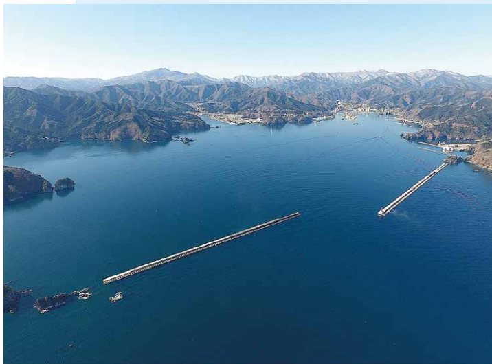
釜石港湾口防波堤
